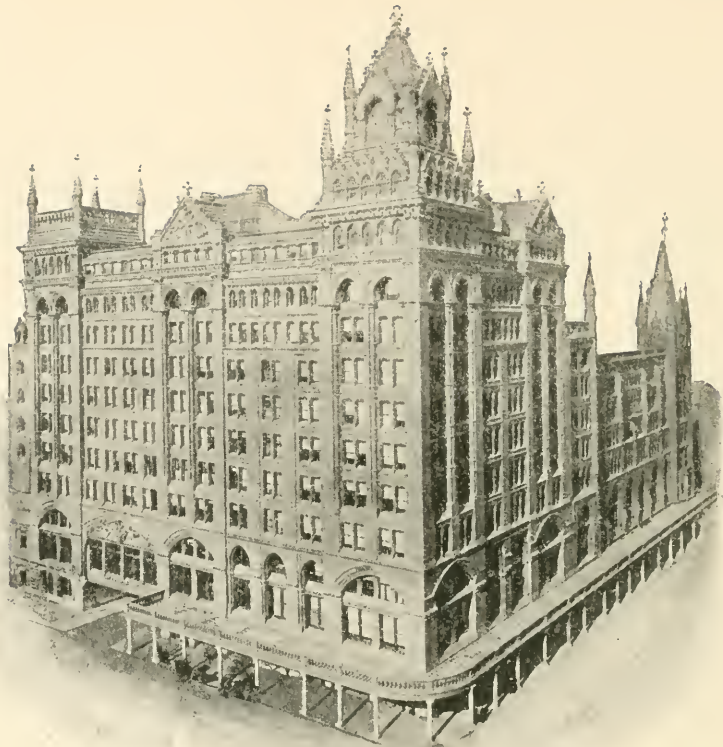
BROAD STREET STATION, PHILADELPHIA.
